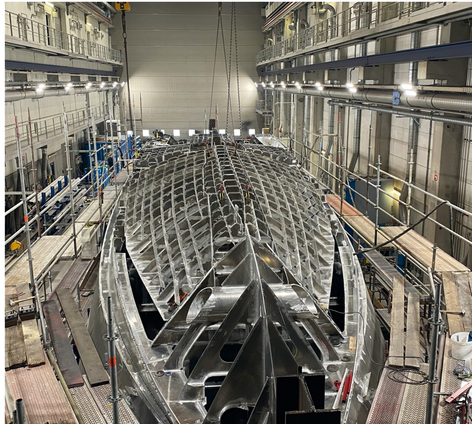
23 m Fast Lightweight Hull (under construction)
